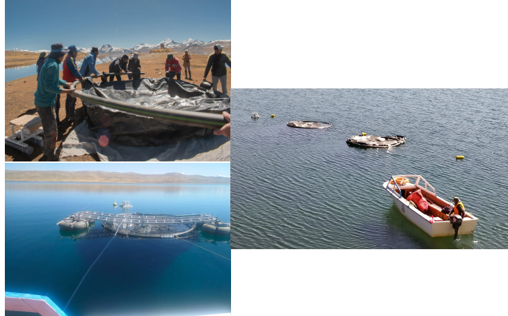
Deployment process of two AQUAMATE bladders at Sibiracocha lake (5000 masl).
